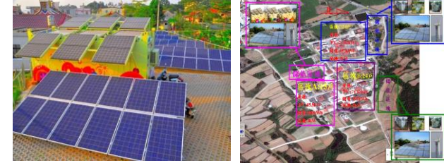
Dongkeng Smart Grid Demonstration Project
